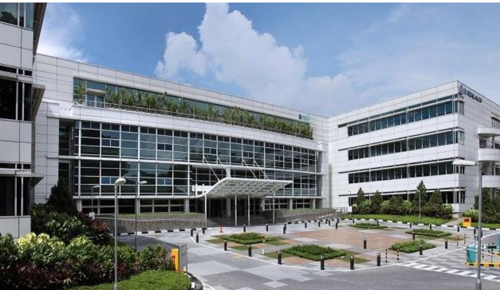
5-storey building with basement carpark
